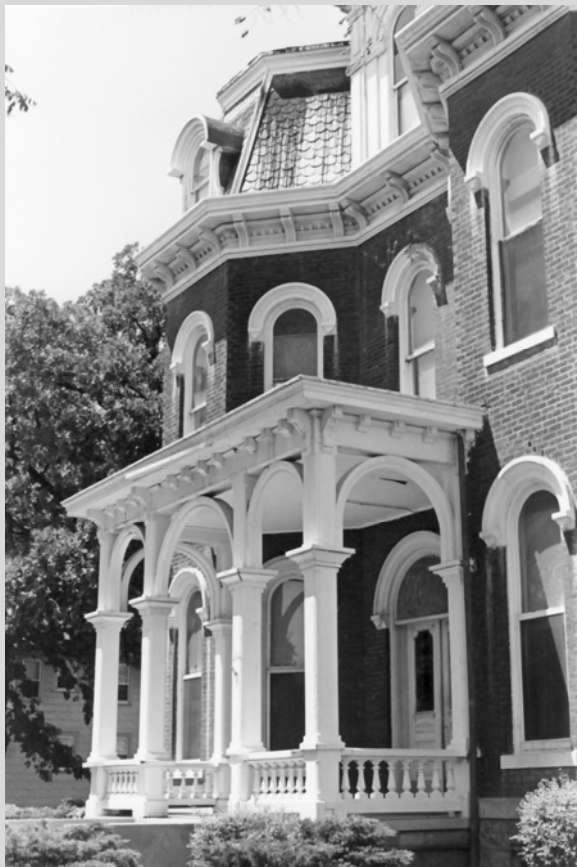
Detail of east elevation looking southwest NSHS H673.5-2375
